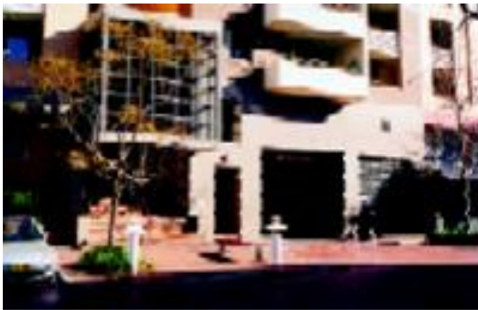
Figure 58: This elevation treats the car park entry as part of the whole elevation. It narrows the width of the entry and defines an opening in proportion to the other facade elements.
